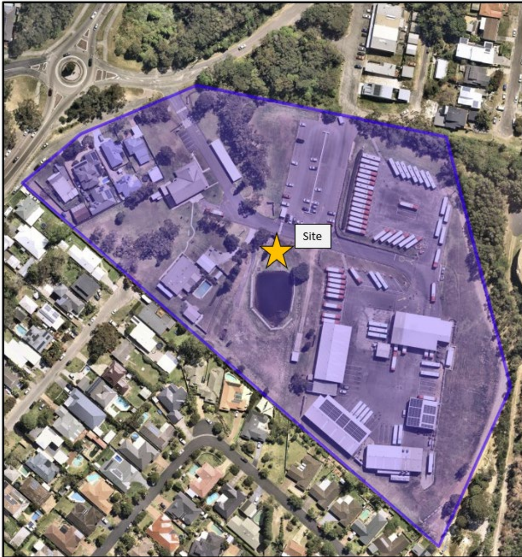
Figure 2.1: Aerial Photo of Site (Nearmap 2022)
